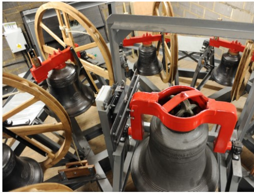
NEW PEAL OF EIGHT IN RADIAL FRAME TOGETHER WITH ELECTRICALLY SWUNG BOURDON AND STATIONARY SERVICE BELL, SOUTH OCKENDON.
